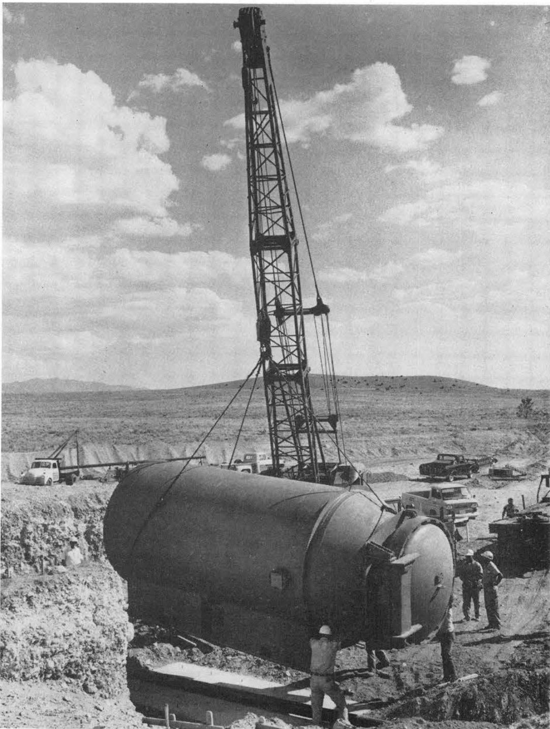
EASY DOES IT — A 37,000-lb. steel firing chamber in Coyote Test Field will be part of a new facility to develop explosive-actuated power supplies. High speed cameras, protected by heavy glass, will record results.
