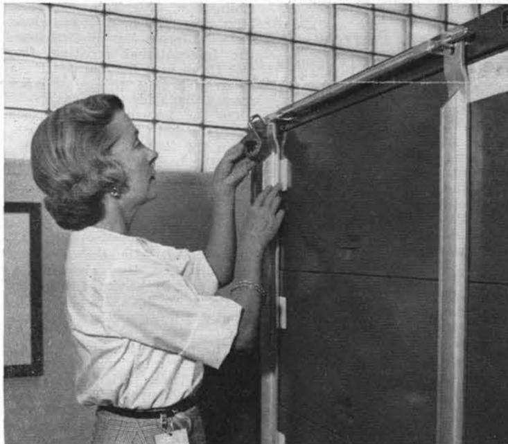
NEW LOCKING DEVICE developed by Floyd D. Norcott and Ralph S. Fox (both 2533) is demonstrated by Justine Bassett (2530). The sliding bar at top of file cabinet eliminates use of one combination lock and saves time. Manufacturer of cabinet has shown interest in incorporating idea.
