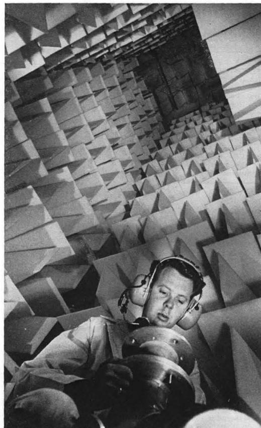
WEDGE-SHAPED batts of foam damp the terrific sound produced by horns at 7300's Acoustic Facility. John Windsor (7324-2) wears headset for protection from ear damage. He can communicate via microphone, earphones with others in building. During test, personnel observe events in this chamber through a multi-pane window from which air has been evacuated. Vacuum kills excess vibrations in window.
