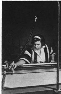
PLOTTING TABLE prepares graph sheet from data cards. The table typifies equipment which speeds up acquisition, increases accuracy of test results. Martha Bullock, of Data Processing Division 7333, adjusts pen assembly on table.
