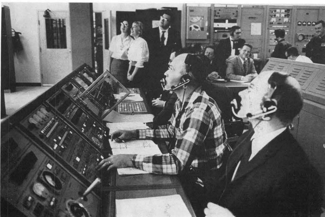
TELSTAR SPEAKS AGAIN — Bell System engineers manning control panels at the Andover, Maine, ground station keep their eyes fixed in the television monitors above them as they see the pictures sent by Telstar after six weeks of silence caused by radiation damage. Daring engineering restored the satellite's operation.
