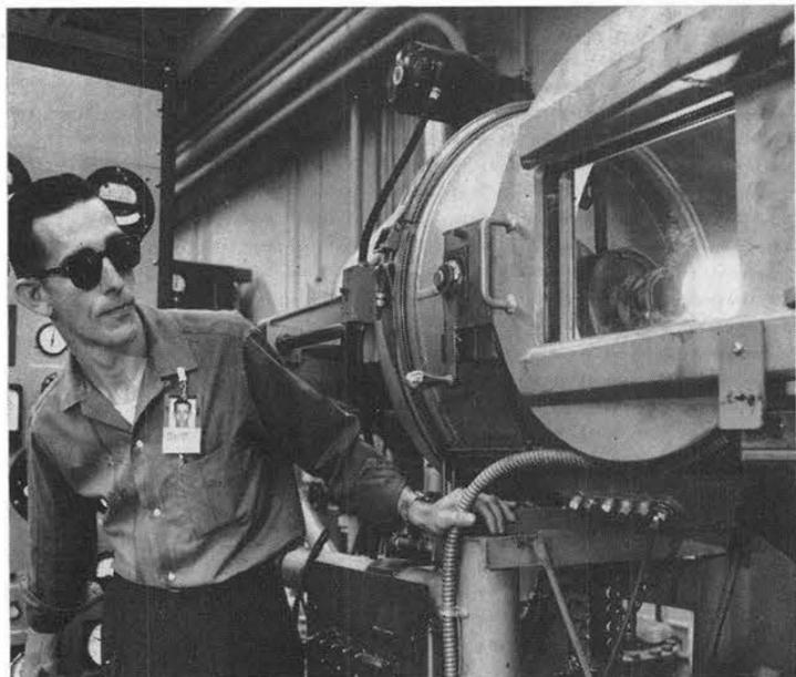
CONTROLS of 120-kw plasma generator are adjusted by James V. Williams (7131-1). Nozzle of plasma generator is visible through window.
