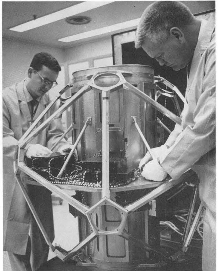
ASSEMBLING logics systems in the test detection satellite frame are W. B. Goldrick (7432-2) and F. E. Thompson, 7432-2 supervisor, right. Holes at the triangular points of the frame will contain LASL-designed X-ray detectors. Solar cells will power the satellite instrumentation.
