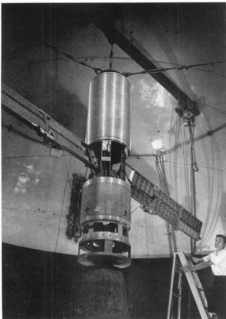
SAMPLER UNIT designed by Aero Design Division 7423 is inspected prior to performance testing in one of the 10,000 cu. ft. vacuum tanks of the Wind Tunnel by Ernest W. Hall (4413), a project designer. The unit is designed to obtain samples of nuclear particles out of the atmosphere from between 230,000 ft. and 100,000 ft. The eight-ft. folding arms of the sampler contain filters and rotate during descent.
