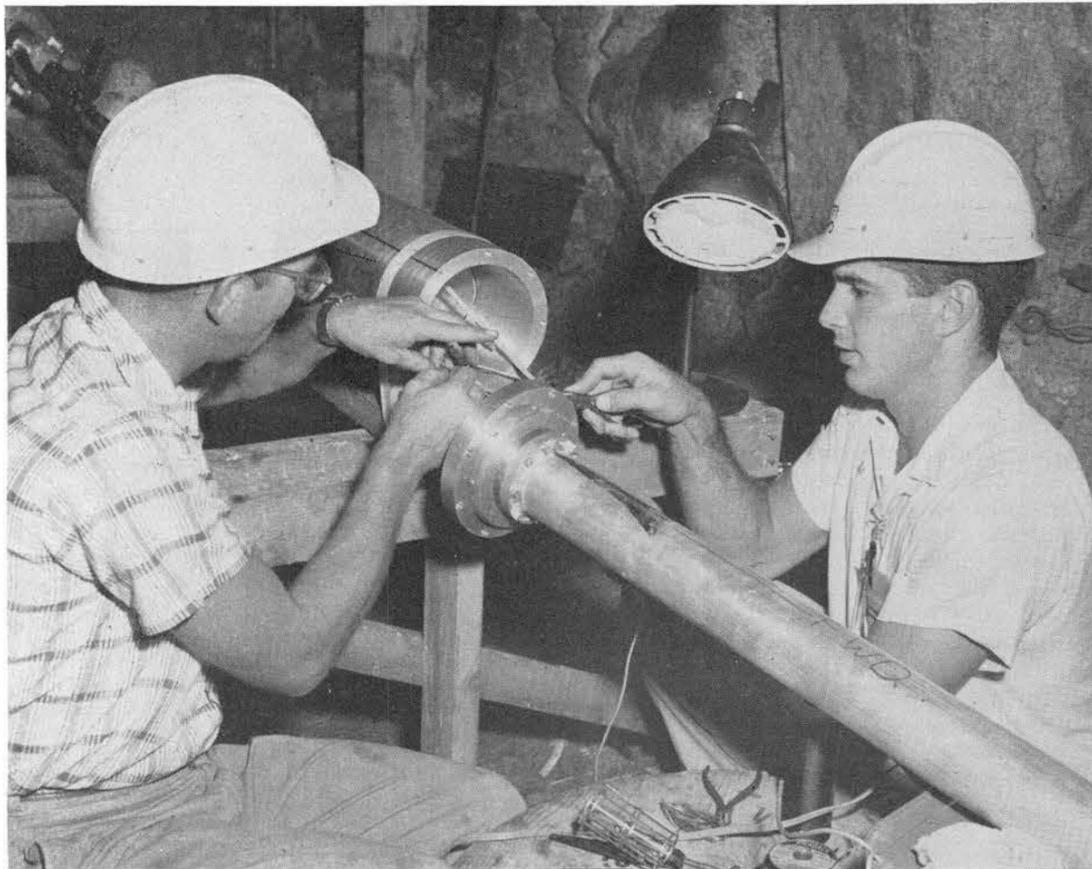
INSTRUMENTATION — L. C. Sandgren, left, and Jim Lohkamp (both 7251) splice cable leading from underground instrumentation canister to trailer located at the site of Project Shoal. The canister contains gauges for measuring velocities, stresses, and strains produced by nuclear detonation experiment. Shot is scheduled for tomorrow.
