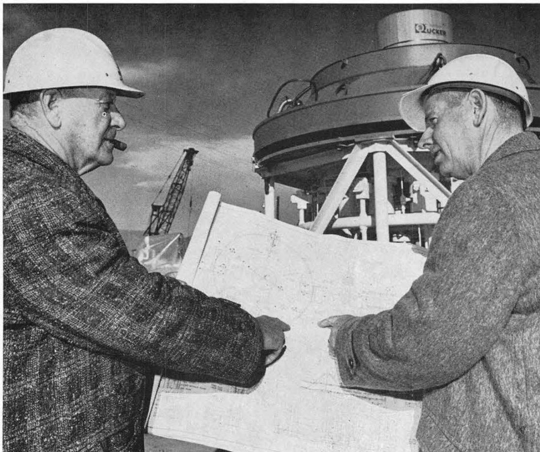
CONSTRUCTION of the new 25-ft. centrifuge in Area III has been a major activity of Plant Engineering Department 4540. Rotating mechanism (in background) was being lowered as Jack Meister, inspector for the contractor, (left) discussed plans with plant inspector R. R. Boyd. Project engineer was R. G. Piper.
