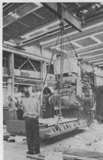
Numerically-Controlled Milling Machine is Installed
