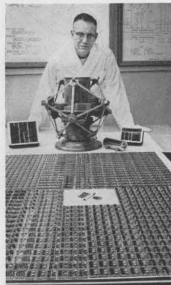
Components for Logics System of Detector Satellite
