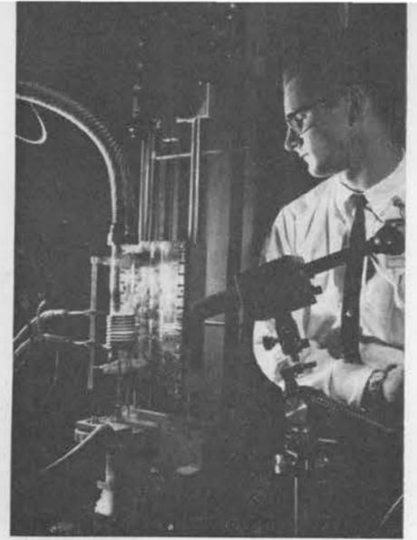
RESEARCH ACTIVITIES of Aerospace Nuclear Safety Department 7410 include special studies of reactor materials at high temperature. Frank Wessling (7411) uses an induction heater and vacuum system to investigate material interactions with graphite. Temperatures reach 5400 degrees F.
