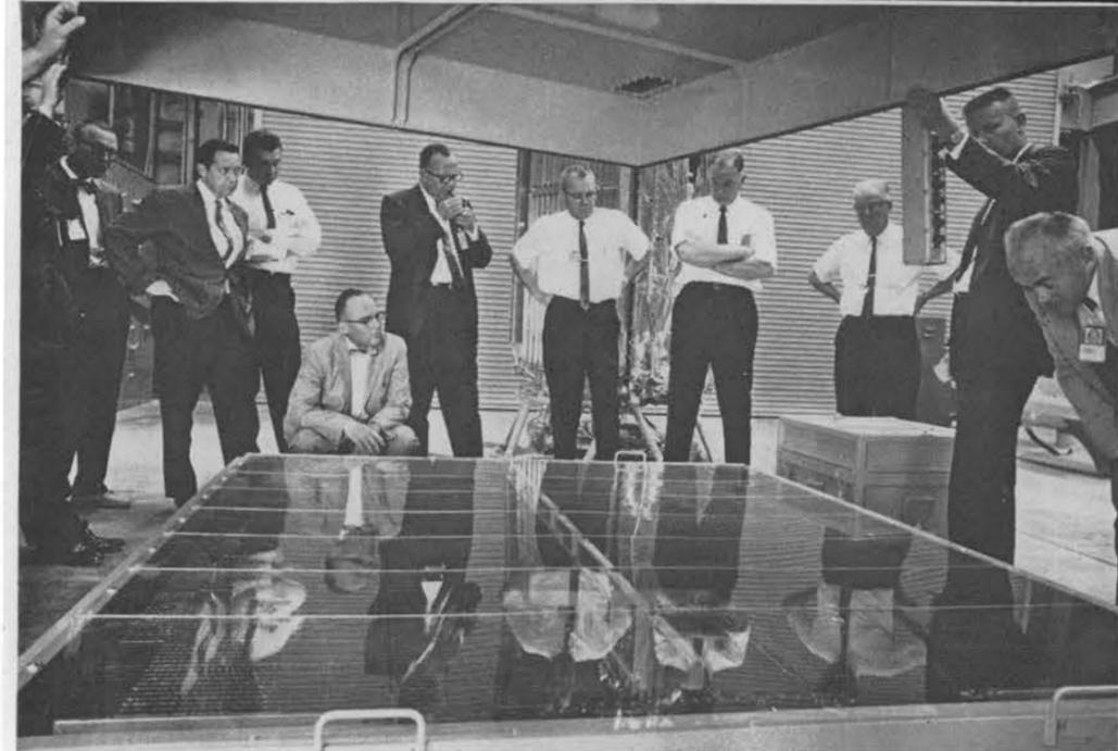
SOLAR PADDLE for OGO satellite, two of which will be carried aboard the satellite, is examined by members of Sandia Corporation's management staff. Each paddle carries a six-by-seven-foot array of photo-voltaic solar cells which will provide the electrical power.
