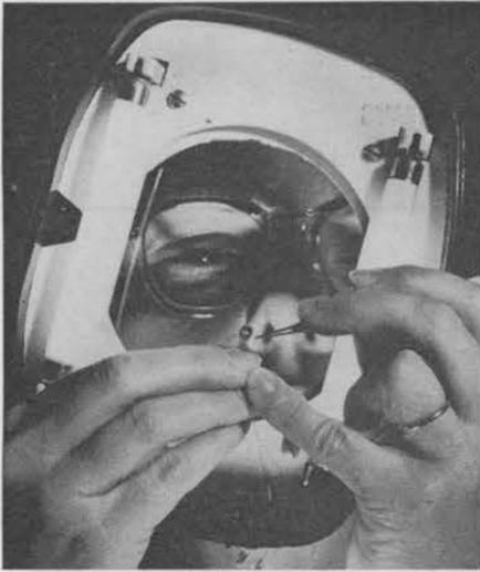
THIS TINY TOROIDAL transformer was carefully wound by hand in Sandia's Transformer Section. It's inspected here under an illuminated magnifier by Helen Agats, who uses tweezers to separate hairlike lead wires.
