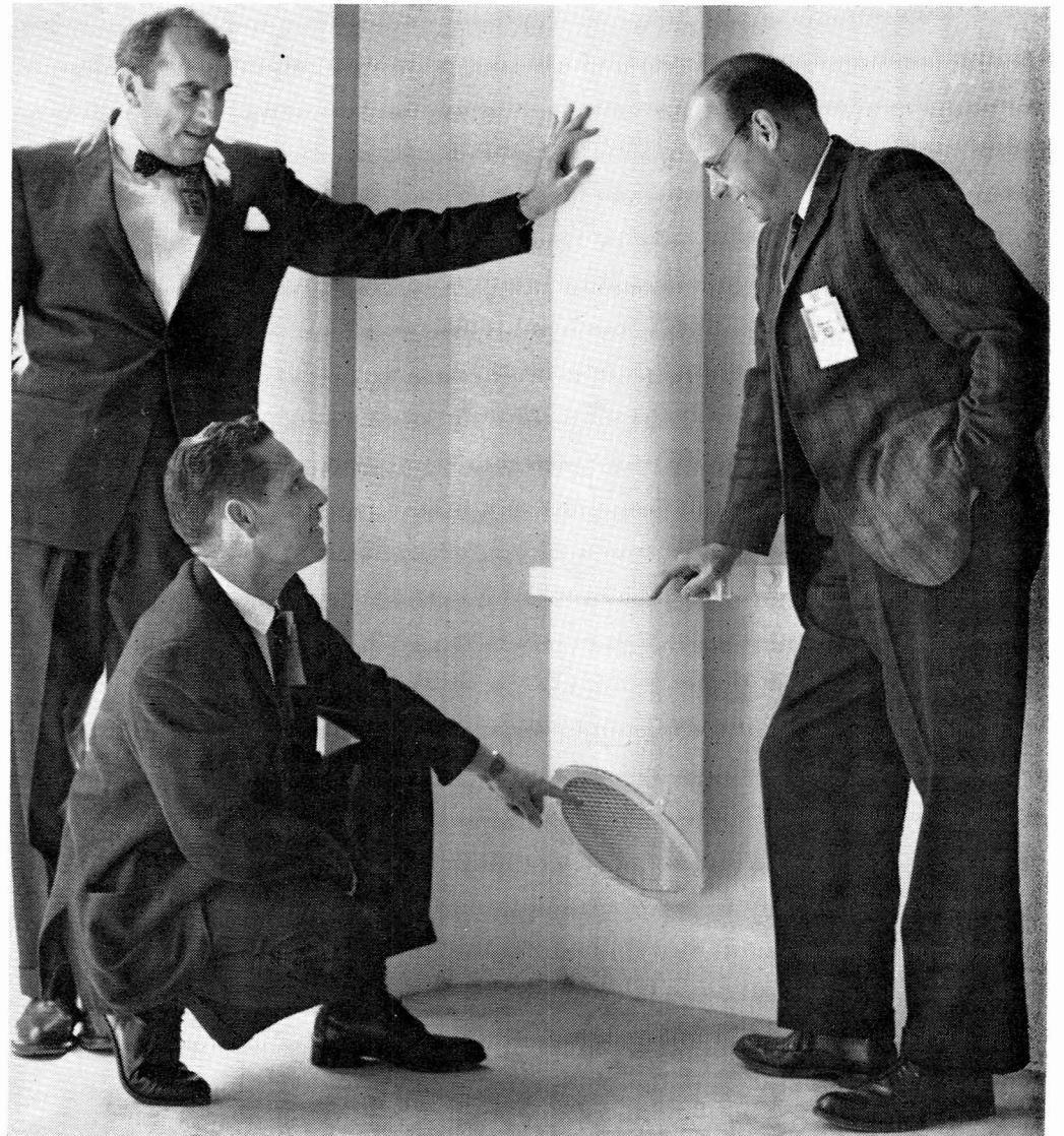
OVERSIZE VENT for exhausting overpressure, gasses, and other HE-detonation byproducts is described by L. R. Myers (kneeling) to F. J. Maloney (left), supervisor of Area 8 Hazardous Test Division, and L. B. Bedinger of Plant Engineering Division. This is one of four similar cells used to subject HE components to specific environments of shock, vibration, acceleration, and temperature extremes. Although components are not intentionally detonated, they are tested in these enclosures so any blast will be contained.
