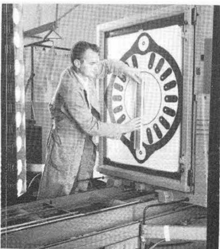
COPY CAMERA—Installation of this large process camera was the last step in consolidating all SCLL photography under one roof. For several years these varied photographic capabilities were housed in different buildings and in temporary trailers around the Laboratory. Putting the camera to use is Ron Johnson.
