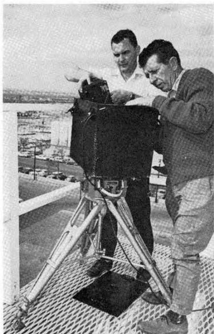
70-mm CAMERA is installed at the Albuquerque Sunport by Clarence Robertson, left, and John Banker (both 7226). The camera will be used in a joint city and county study of air pollution. It will make photographs every five minutes.
