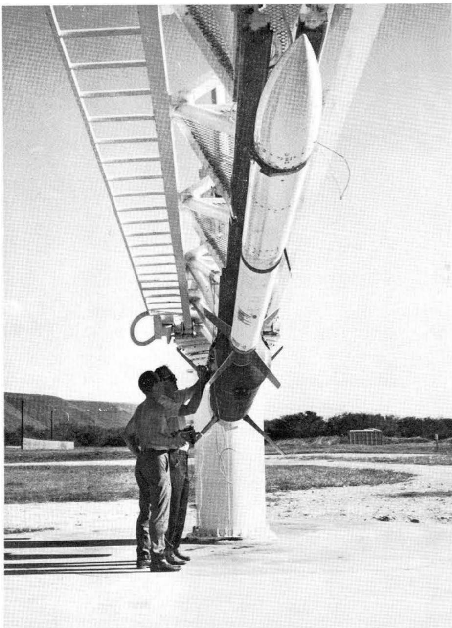
CHECKING FIRING CIRCUITS are Roger Gelder and Jim Malloch. The Nike-Cajun rocket is assembled with the payload on the launcher and almost ready for firing. The launcher can be raised to any angle and aimed for the proper rocket trajectory.
