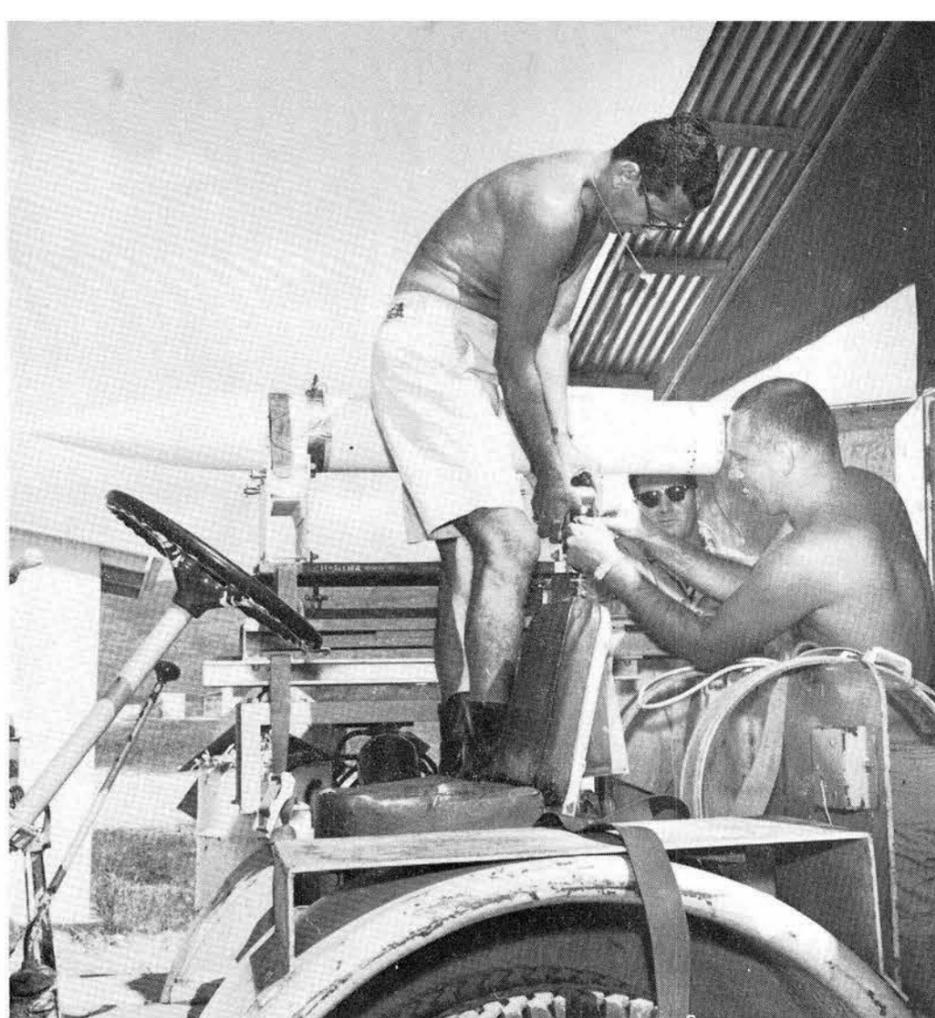
ROCKET PAYLOAD, containing the deflated spheres which will be ejected at high altitudes, inflated, and tracked by radar, is readied at the "screen room" at Barking Sands. From left are Jim Strascina, Bruce Barth, and Lee Stone.
