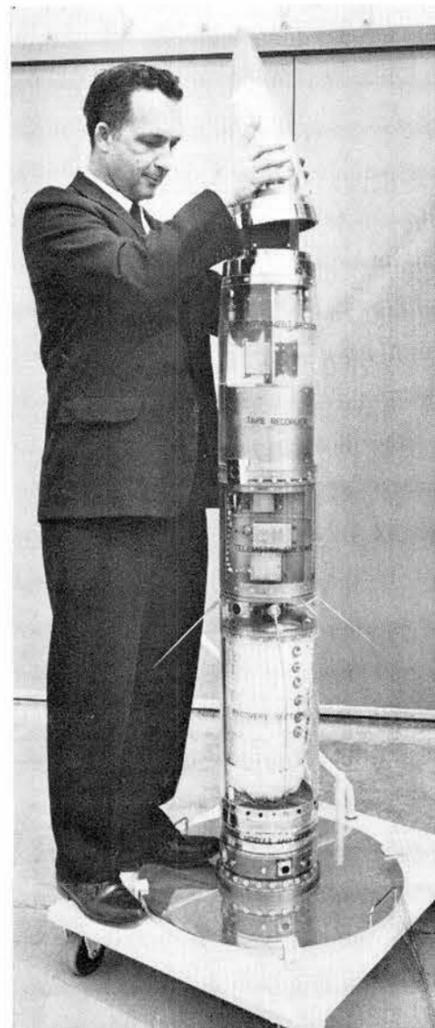
**TYPICAL PAYLOAD** — Nitehawk 9 model payload section is examined by W. C. Womack, project engineer for the sounding rocket system. Instead of the conventional metal casing, this demonstration section is covered with plastic to show the location of typical payload components which are labeled for briefing purposes.
