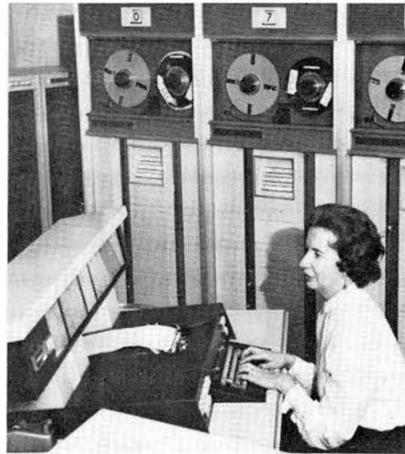
OPERATING Control Data 3600 Computer recently installed in Bldg. 912 is Mrs. A. E. Crow (8144-3). The new facility will centralize all of Livermore Laboratory's computer needs.
