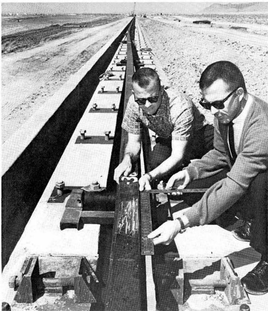
CURVE OF THE RAIL will disappear when the rail is positioned between the bolts of Sandia's new 5,000-ft. sled track in Area III. Inspecting a newly welded rail joint are Bill Kampfe (left) and Marv Timmerman (both 7344). The 39-foot rail sections are welded using a pressure-fusion process and then ground smooth. The new track should be operational in November 1966.
