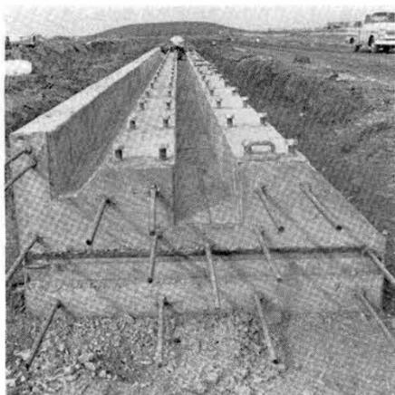
SLED TRACK RAILS will be secured by bolts and clips. The troughs (left and center) will permit water braking by probes from monorail sleds.
