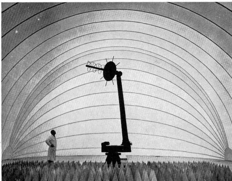
RADIATION PATTERN MEASUREMENT TEST of a four-turn helix antenna is checked by Ronald D. Bentz (1424) in an inflated nylon "balloon" section of Bldg. 9970. The antenna is mounted on a model pedestal which is remotely operated from a console in an adjoining room. The pyramid-shaped foam plastic (lower foreground) is used to eliminate reflection of radio waves.
