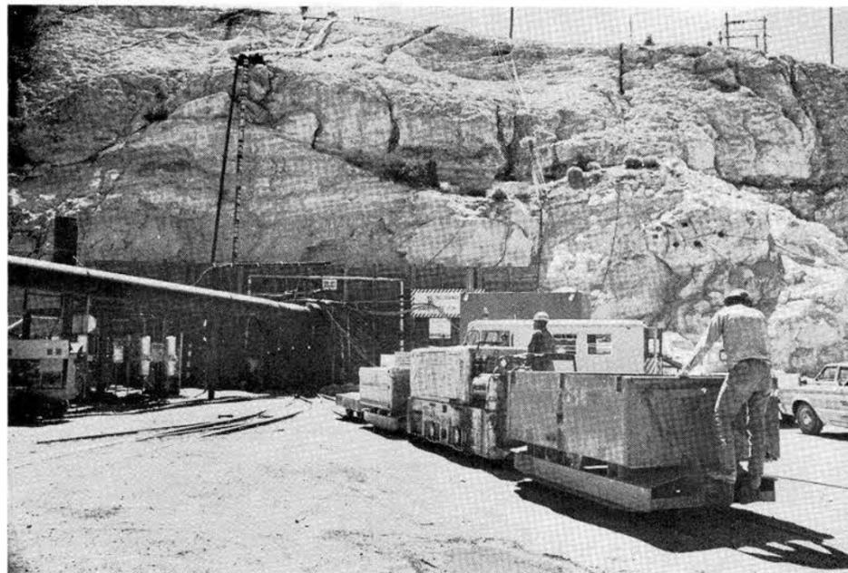
ENTRANCE to a tunnel site prior to an underground test is scene of massed activity as miners shuttle equipment into the tunnel and engineers check cables and instrumentation. Large pipe leading into the tunnel is part of the Sandia-designed air filtration system.
