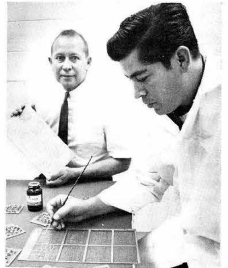
ART CORDOVA (left), supervisor of Sandia's Printed Circuit Shop, displays a circuit board covered with silver paint to tie in conducting elements prior to electroplating and cleaning. Art's spray method, combined with preparatory processes, saves time and money over former method of hand painting the connections, demonstrated by Richard Chavez (4233-3).
