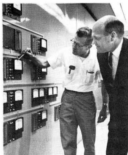
STATUS OF CITY'S WATER is checked by William P. Walker (left), Water Division Operations superintendent, and Commissioner Kinney. The panel is in the City's Water Operations Central Control building at 2629 San Mateo, N.E. Information such as water levels in the reservoirs and water pressures at the various sites throughout the city is shown on the board's instruments. There are a total of 86 wells, 29 reservoirs, and 26 pumping stations in the water system.
