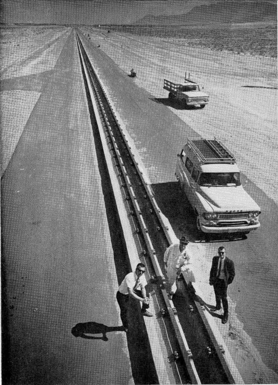
NEW 5000-FOOT SLED TRACK in Area III has exceeded design specifications. Some 75 rocket sleds have successfully been fired at the new facility. At left is Marv Timmerman who prepared the design specifications for the track. In the center, marking the water trough and 22-inch gage of the track, is T. R. Arrington. At right is Bill Kampfe, track project leader. All are in Division-7344.
