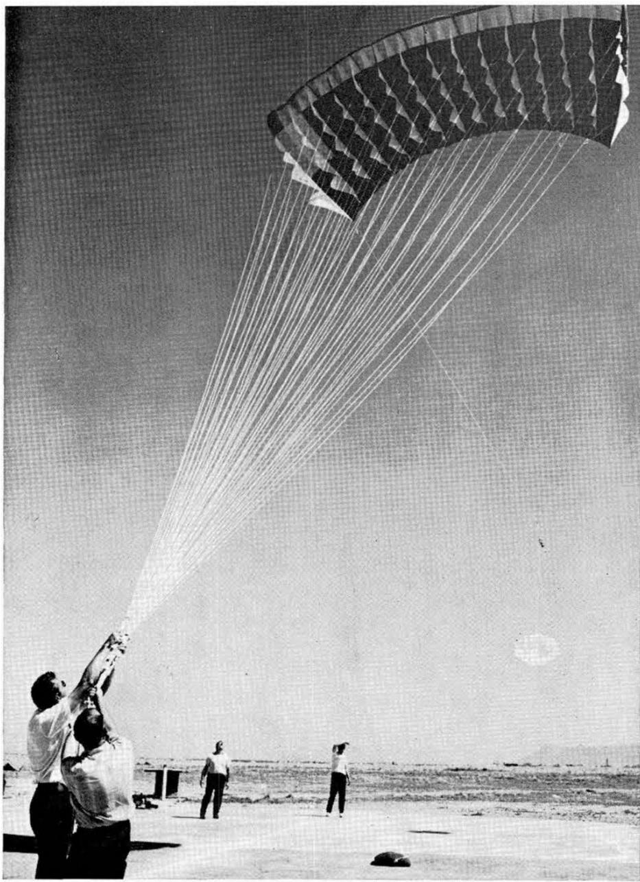
KITE-LIKE, a Para-Foil is launched by Division 9324 personnel during a test in Coyote Test Field. The system when tethered with a cable provides a stable "sky-hook" for instrumentation cables. In free flight, the Para-Foil is combined with an automatic homing system which brings rocket payloads down to a ground station transmitter.
