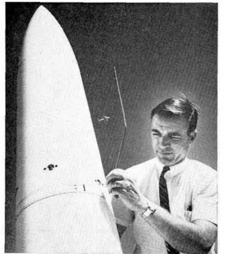
ATTACHING TELEMETRY ANTENNA to a Sandhawk payload is Les Luehring (9224), project engineer for the new single-stage rocket system. The payload is 13 inches in diameter and 7 1/2 feet long.
