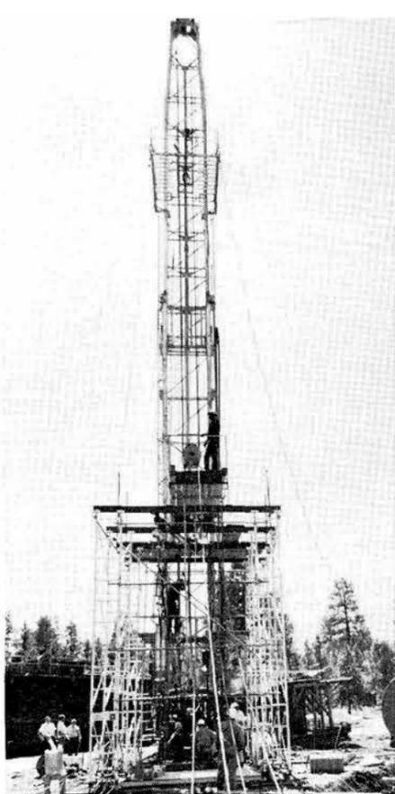
HEAVY DUTY CABLES—16,000 feet of it—run from remote recording trailer and down the drill hole to the buried Sandia seismic instruments. The Gasbuggy site is in the Carson National Forest, 50 air miles from Farmington.
