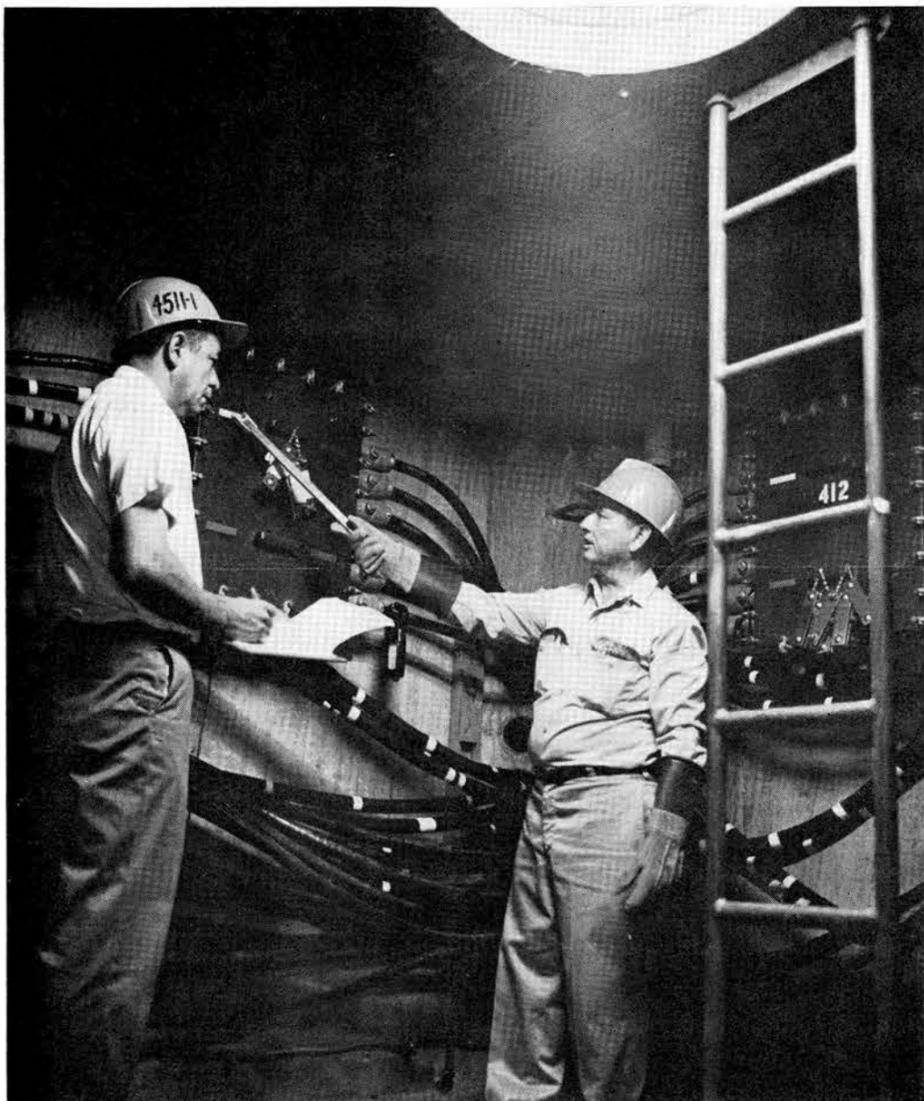
INSIDE A MANHOLE, Henry C. Sisneros reads off the correct procedure while Louis J. Price (both 4511-1) checks the circuit load of a power line.
