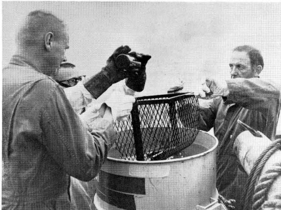
SAFELY RECOVERED from the ocean floor, two SNAP 19 fuel capsules are examined by (l to r) Bob Luikens (9521), Bill Gaines (3312) and John Adams (AEC/ALO) prior to shipment in a special container to Mound Laboratories. The two capsules, valued at \$700,000, survived rocket launch abort and almost six months under the sea in good shape. The cases around the plutonium 238 were undamaged.
