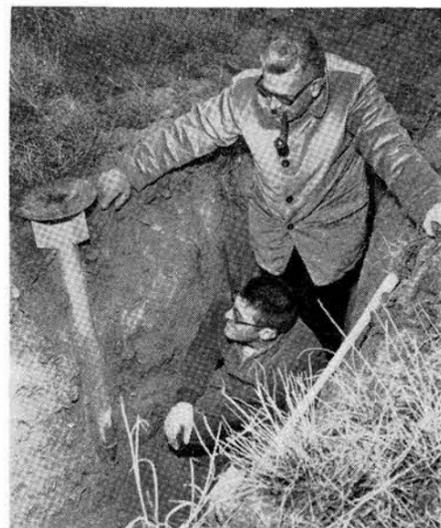
MAN, DIG that crazy postholer! Penetrometers designed and developed by Terradynamics 9327 make a nice, neat hole in the ground but serve a more useful function as a means to obtain remotely the soil data necessary to establish airfields in forward or hostile areas. John Colp (standing) and Ed Villella (both 9327), examine one of the earth penetrating instruments after test drops made at Sandia recently.
