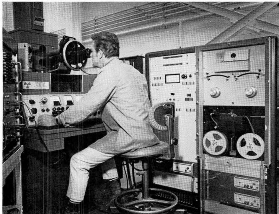
**SIX KW ELECTRON BEAM WELDER** is operated here by **Jim Taylor** (4221-5). Large vacuum chamber behind controls can contain items from the very small to about 18 inches in diameter. Welding
