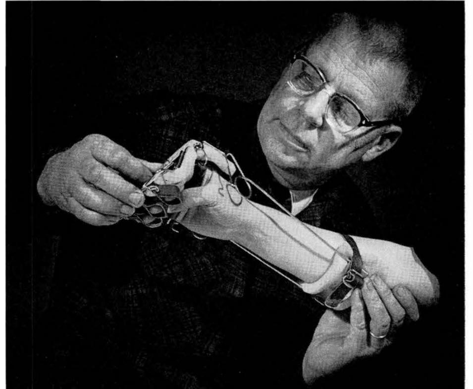
ORVAL WALLEN (8243) adjusts one of the medical braces he made in his spare time for the patient of a local doctor. The braces, of spring steel with handsewn padding and supports, help restore muscle deterioration or straighten deformities.
