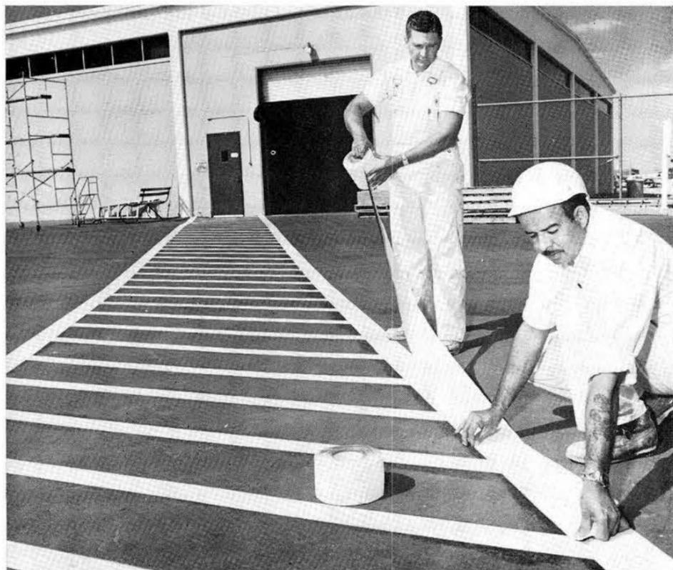
PAINTERS Wayne Phelps, left, and Ted Ortega (both 4513-3) demonstrate ease with which new metal tape can be used to mark Sandia crosswalks and parking areas. Use of the tape instead of conventional brush painting will save the Laboratories \$8200 annually.
