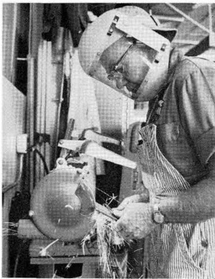
PROTECTION from grinding wheel accidents is afforded by using tools properly and wearing the appropriate safety device such as a face mask. Dale Easton (4512) demonstrates.
