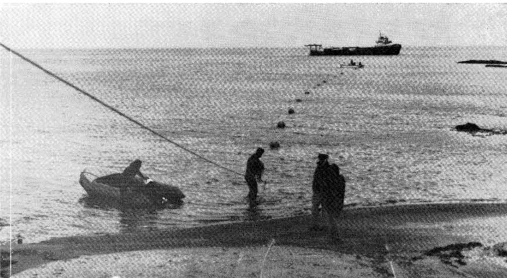
**CABLE** from underwater instrumentation to recording trailer park is being strung by a crew from the "Sea Tender." The instruments recorded shock wave in the sea around the island resulting from the Milrow detonation.
