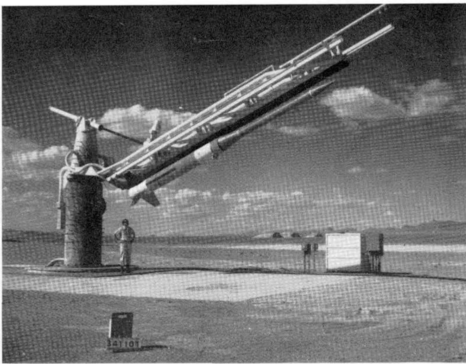
LAUNCH ANGLE of 20 degrees is used for new high velocity, low altitude rocket test vehicle designed by Sandia. Gary West (7250-A), test project manager, inspects the two-stage vehicle on launcher at Tonopah Test Range.
