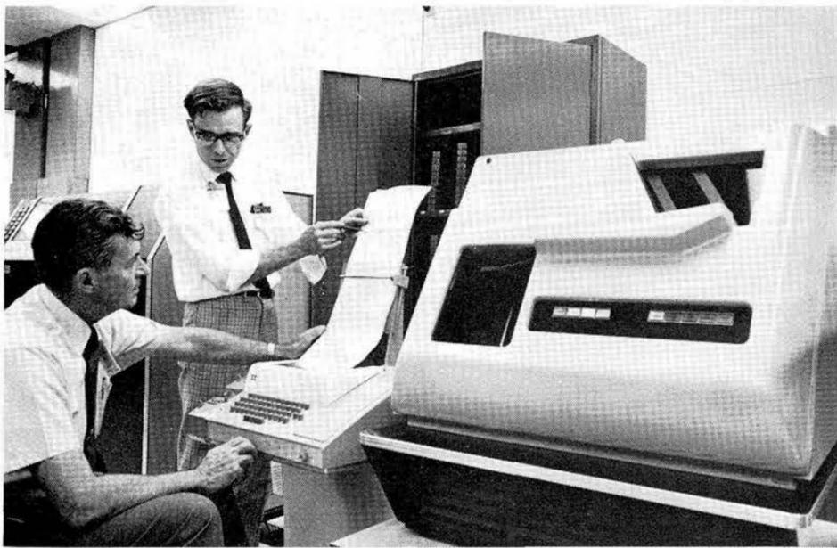
SYSTEMS CHECK of the new PDP-10 computer is made by systems analysts Phil Eyre, left, and Larry Lane (both 9421). The new computer is now "on-line" and operating with 36 remote terminals throughout the Laboratories.
