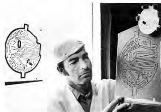
**STAGES** in the photochemical production of a printed circuit board are displayed by Jac Constant (4221-1). At left is a film negative of the master drawing, in the center is a template made from photopolymer, and in the upper right is a printed circuit board ready for installation of components. The new technique using photopolymers and chemical etching is described in the accompanying article.
