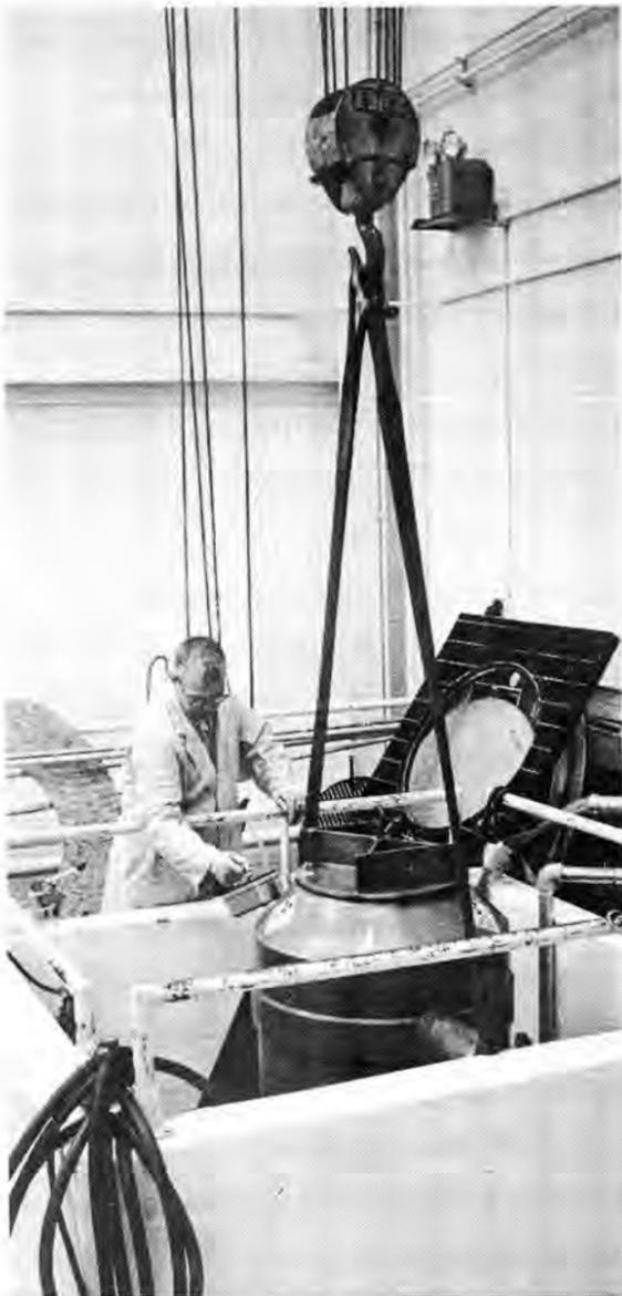
SPECIAL SHIPPING CASK containing four fuel elements from Sandia Engineering Reactor is raised for radiation readings by Health Physicist Charles Berglund (3311). Work is being done in connection with final shutdown of reactor after many years of service.
