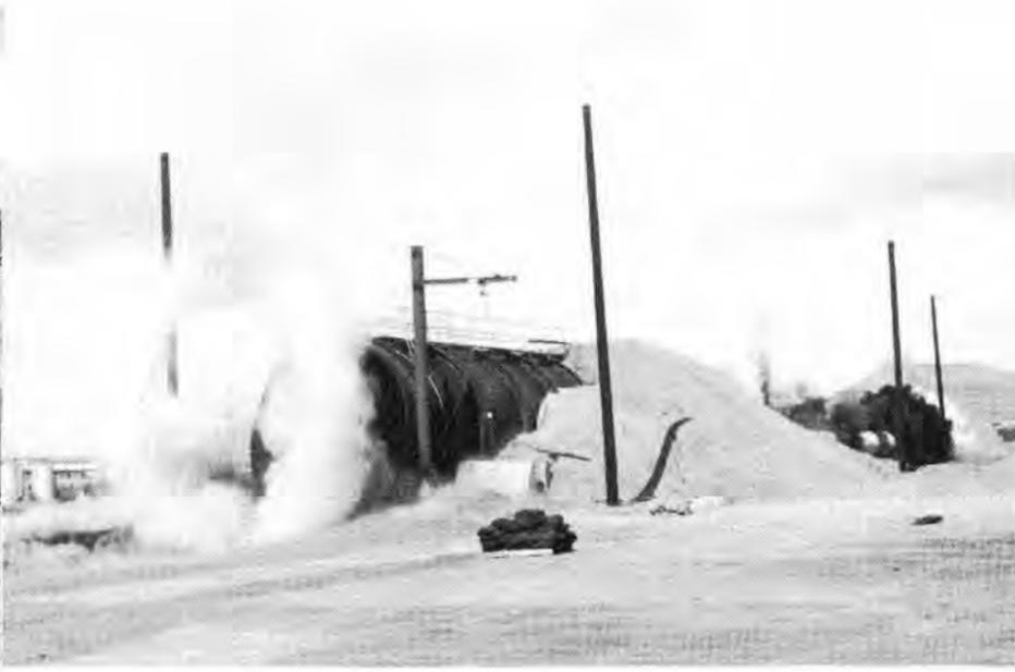
TEST SECTION of Sandia's new shock tunnel is checked by Manuel Vigil (9322), project engineer for the facility. The end of the 19-foot-diameter section is cut at a 75 degree angle to accommodate large test items which are
