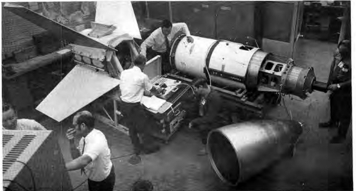
SYSTEMS CHECK is conducted on Strypi rocket which contains Sandia-designed system to jettison Recruit booster rockets after burnout. The two boosters are mounted on tracks, one of which is visible between the two fins on the lower left.
