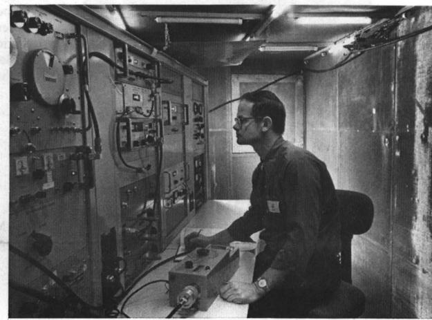
USING THE primary lab's two-pressure humid atmosphere generator, Bill Huff calibrates instruments which measure relative humidity.
