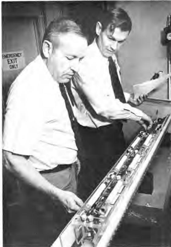
PROTOTYPE drilling head that employs shocks generated by electrical detonations was assembled from "off the shelf" components to prove feasibility of the concept. Gordon Harvey (5724) and Bob White (2315) check the unit.
