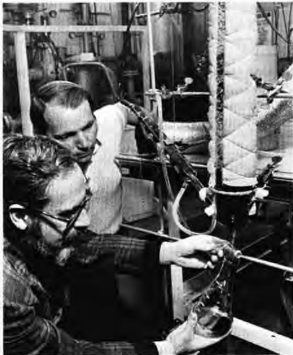
USING LAB APPARATUS, Charlie Arnold (5811) and Dick Curlee (5843) simulate oil shale *in-situ* processing. The asbestos-covered glass tube contains oil shale rubble which has been ignited at top. As the rubble burns down, oil collects at bottom of tube.
