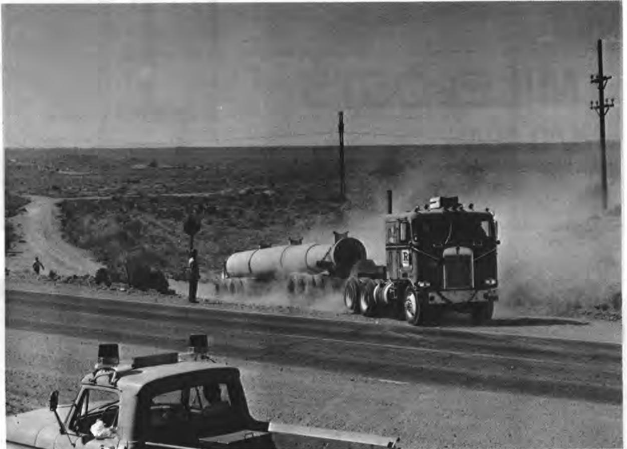
59 TONS of gun barrel leave Sandia for Oblivion. With an equal-sized partner, it served as a test facility in Area III since the mid-fifties. Originally from the Naval Gun Factory, the 45-foot barrels were bored out to a 26-inch diameter and used both as a pressure vessel and as an explosive gas shock tube. Subroc missile, now in the fleet, was its biggest test. Here it's a test of traction and power as a contractor/purchaser eases the big barrel across Tijeras Arroyo.
