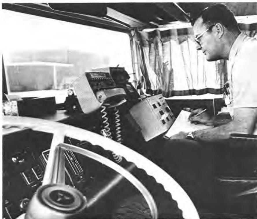
J.T. "THEE" WHEELIS (1739) with message entry unit located in test vehicle. Location and status of vehicle is given by dialing various numbers on the display panel of the message entry unit. Located on dashboard above the unit is a radio telephone, transceiver control and signal strength meter.
