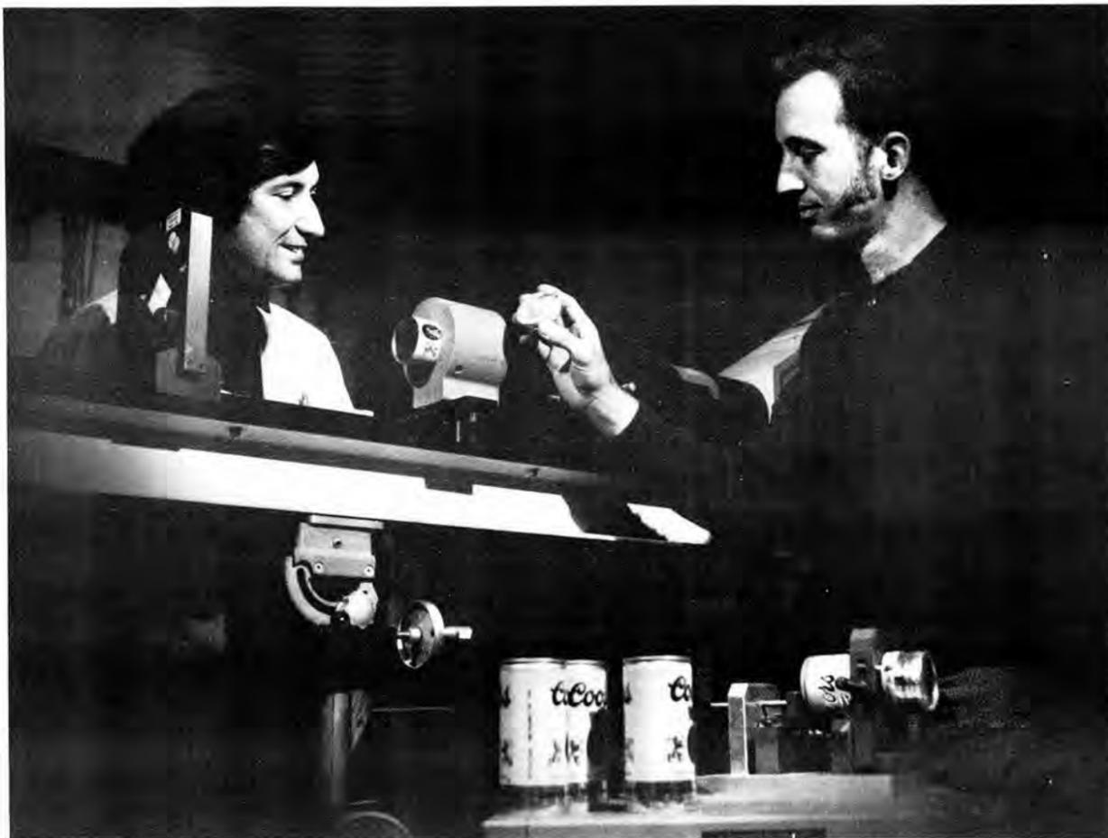
COLLAPSED ALUMINUM BEER CAN is examined by Art Van Hook (8156), right, and Gene Neau (8416) after the can was used in the fast shutter system they developed to eliminate rewrite problems inherent in high speed cameras.
