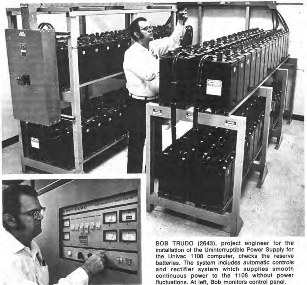
BOB TRUDO (2643), project engineer for the installation of the Uninterruptible Power Supply for the Univac 1108 computer, checks the reserve batteries. The system includes automatic controls and rectifier system which supplies smooth continuous power to the 1108 without power fluctuations. At left, Bob monitors control panel.
