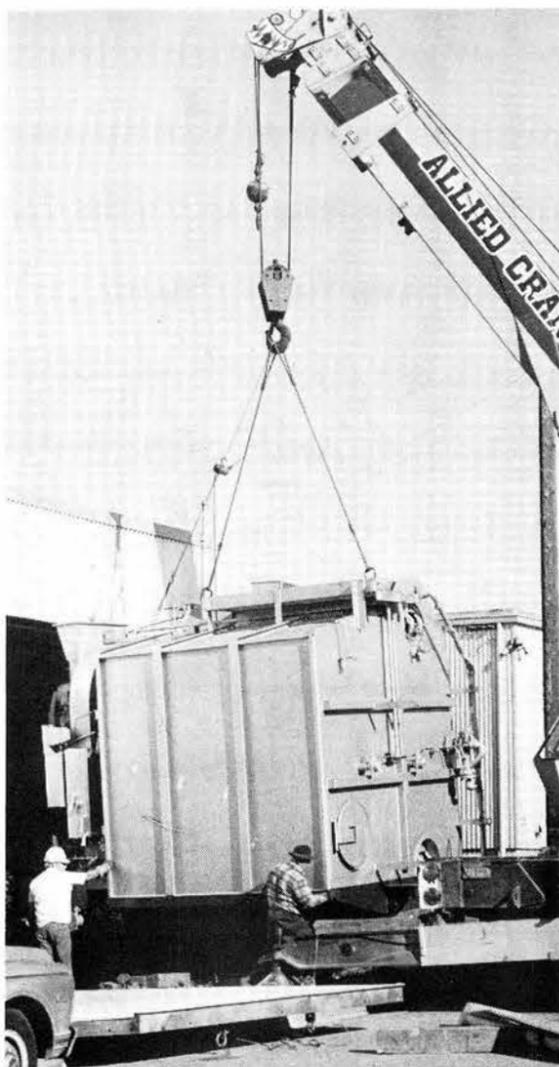
SIXTEEN TONS, and what have you got? A new 16-ton boiler for the steam plant, that's what. Installation provides additional capability, serves as backup to existing boilers.
