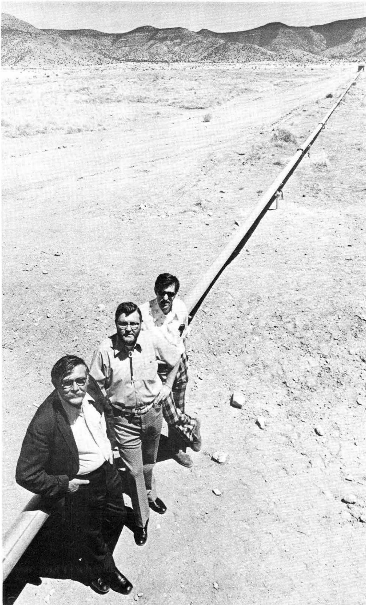
MILE-LONG VACUUM PIPE encloses laser beam, heart of the largest and most sensitive strain seismometer ever designed, operating in Coyote Canyon. From left are Ben Benjamin (1123), Wendell Weart (1140) and Doug Gabin (1111).
