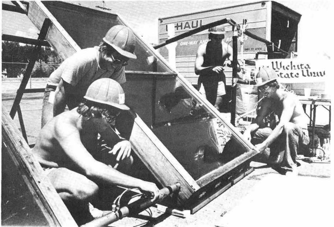
WICHITA STATE solar collectors are designed to provide space heating.
